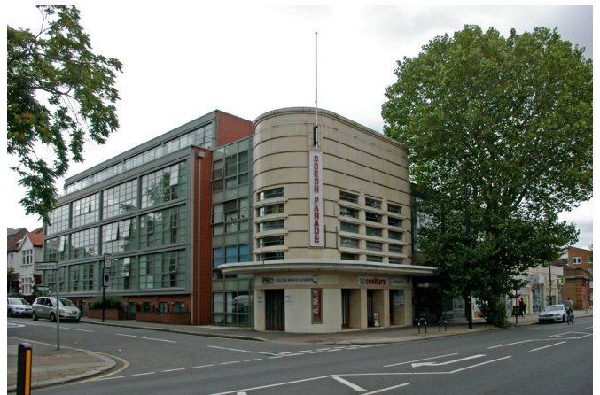
Former cinema, London Road
