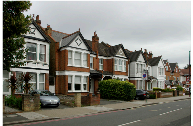
East side of Thornbury Road.
