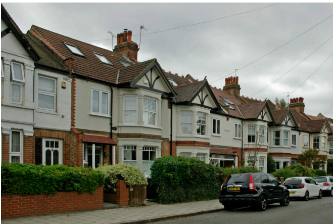
Ridgeway Road between College Road and Highfield Road.
