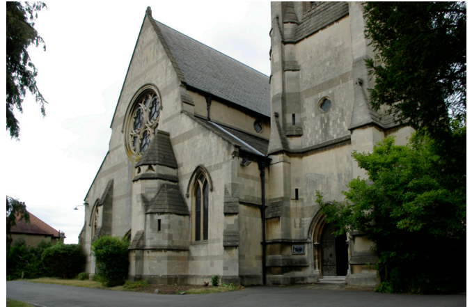
St Mary's Church, front entrance and west elevation.
