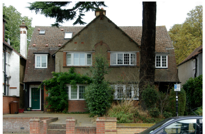
East side of Thornbury Road.
