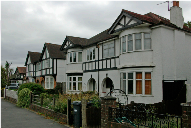
Great West Road between Osterley Road and Ridgeway Road.
