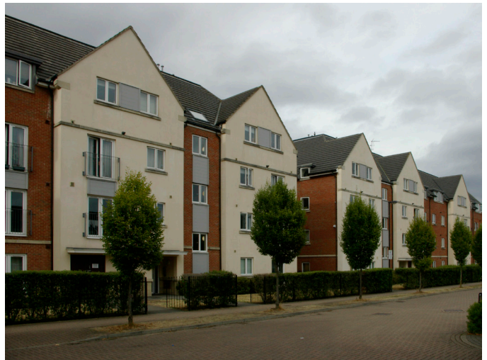
Brunel University site redevelopment, Academy Place.
