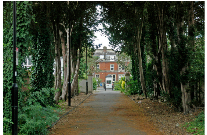
View west along the footpath from the Lodge to Spring Grove House.
