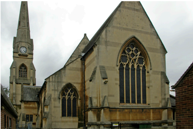
St Mary's Church, rear/east elevation.
