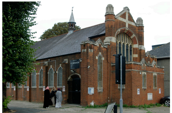
Former church, Thornbury Road
