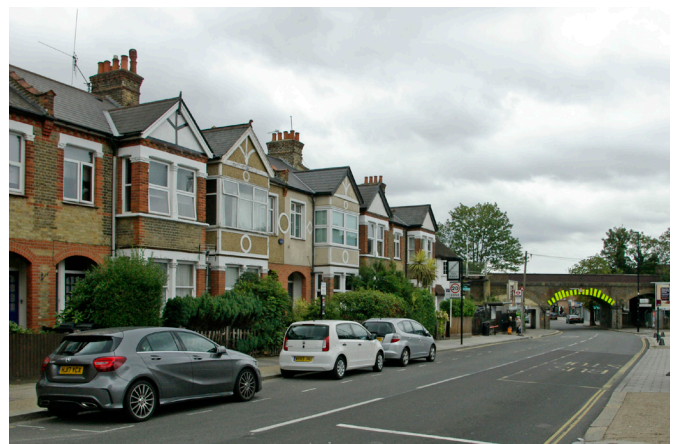
St John's Road and railway bridge.
