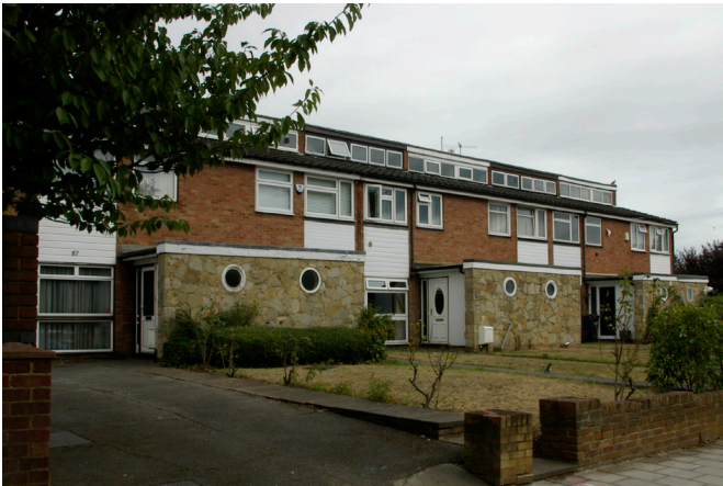
Junction of Thornbury Road and Moreton Avenue.
