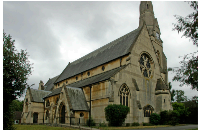
St Mary's Church, north entrance and north and west elevations.
