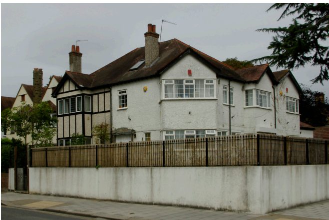
Locally listed houses, corner of Thornbury Road and Church Road
