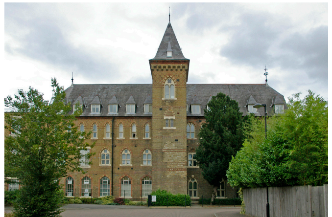
Lancaster House (Grade II), west elevation, Borough Road.
