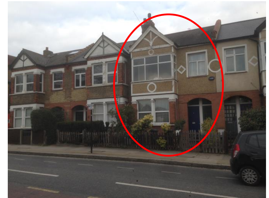
Figure 14: Heavily altered terrace to the east, with a series of remodelled bay windows circled. Source: Site visit (February 2016).
